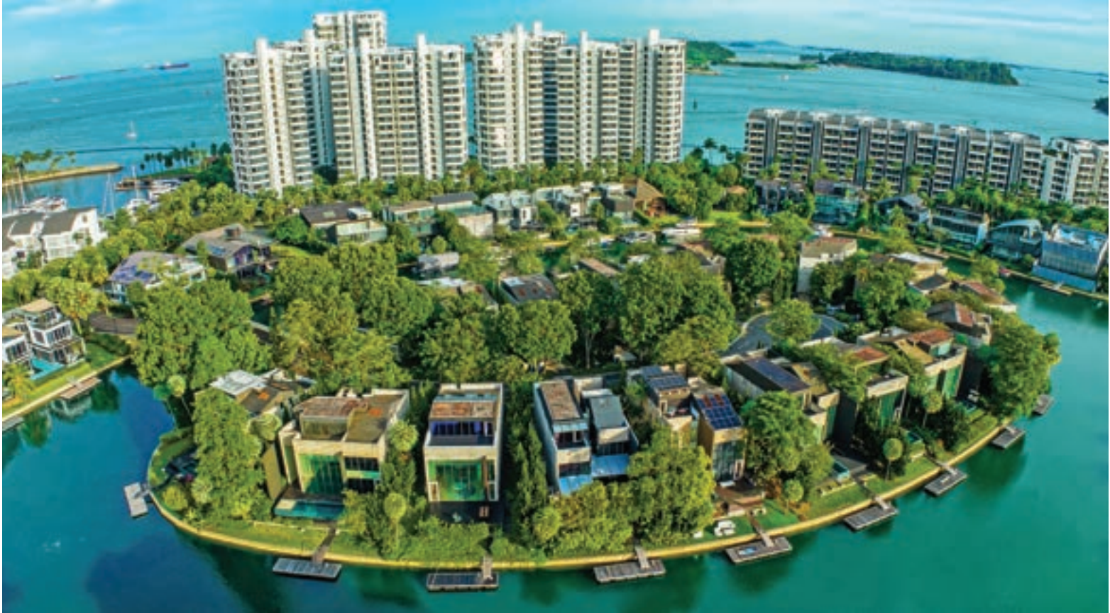
The reclamation of Buran Darat added about 86 hectares to Sentosa's eastern shore, allowing for the addition of new residences in land-starved Singapore, and a host of ultra-luxe developments that elevated Sentosa's branding.
